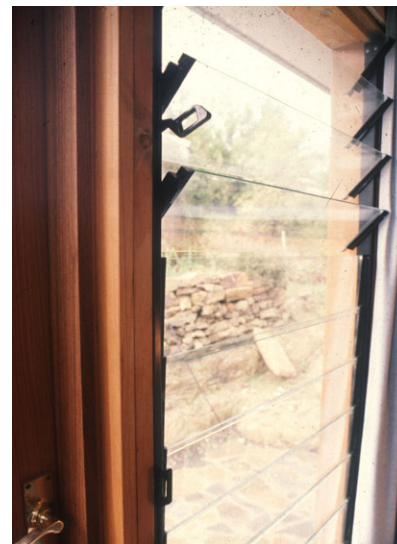
Bedroom louvre windows ("Breezeaway"). Black anodised aluminium on fire-salvaged cypress frame, polypropylene blade clips and 6mm glass blades. External fly screens removed for winter.
