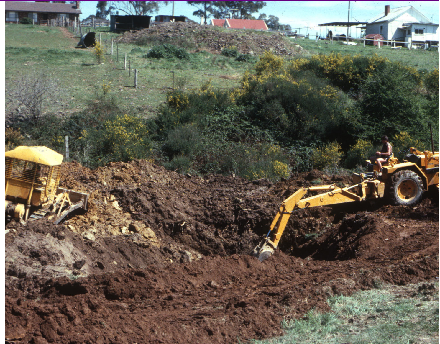
Construction of geese pond September 1987. Backhoe is excavating mixed topsoil/fill to form toe of wall, D3 bulldozer pushing clay into core trench.
