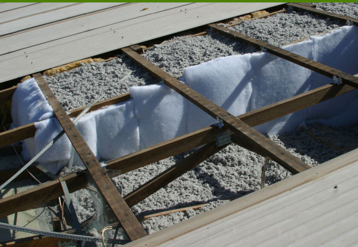
Cellulose loose fill insulation 125mm deep in flat laundry ceiling (front) west bedroom and clerestory cathedral cavities (behind) with polyester batts (R 1.5) on vertical plaster and mudbrick connecting walls prior to fixing of foil sarking.
