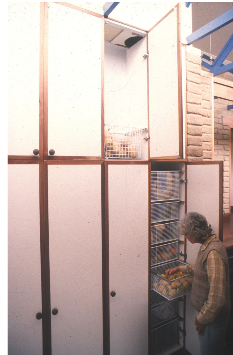
Su opening sliding wire baskets in four doored cool cupboard. Open top door shows half section of 300mm metal exhaust flue pipe. Larger opening at base allows flow of cool air from below timber floor. Grocery and broom cupboards at lower left, bottled preserves upper left. Cupboard doors are made from melamine coated chipboard with blackwood frames giving a flush fitting and easily cleaned door with minimal gassing off of chipboard glues.
