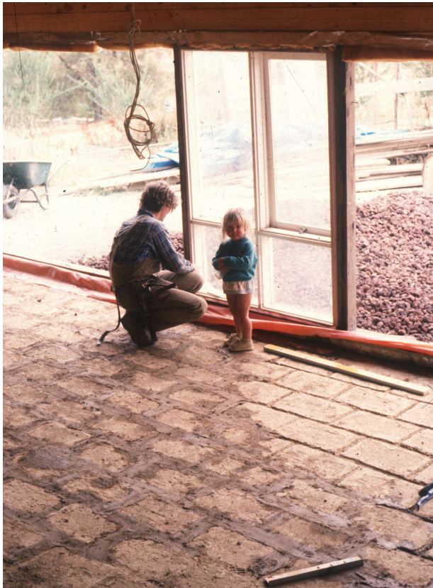
David and Oliver (18 months) fixing second hand north window glazing. Mudbrick floor with first layer of mud/cow manure grout dry and rammed (right) and second topping grout (left)
