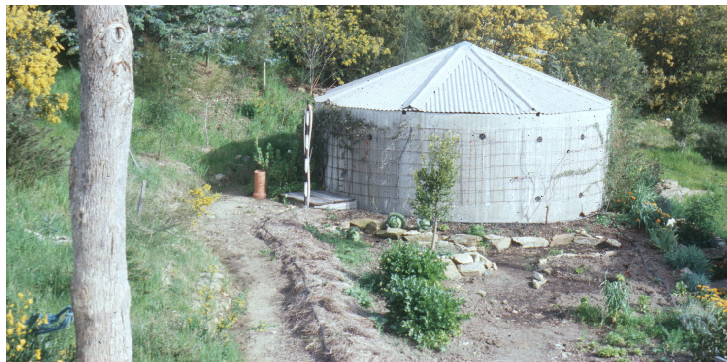
Concrete header tank (42,000l capacity) at highest practical point on property installed 1986 (photo 1992). Sight gauge at left shows water level. Wheelbarrow path/table drain diverting seepage and runoff from cut slope away from housesite. Tank terrace garden ready for spring planting in foreground. Cut slope, screen plantings in background.
