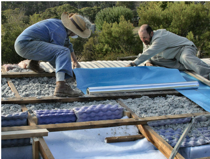
Su and Tony Soccio unrolling foil sarking over roofing battens. Note cardboard apple packing sheets used as baffles to contain cellulose in insulated section.
