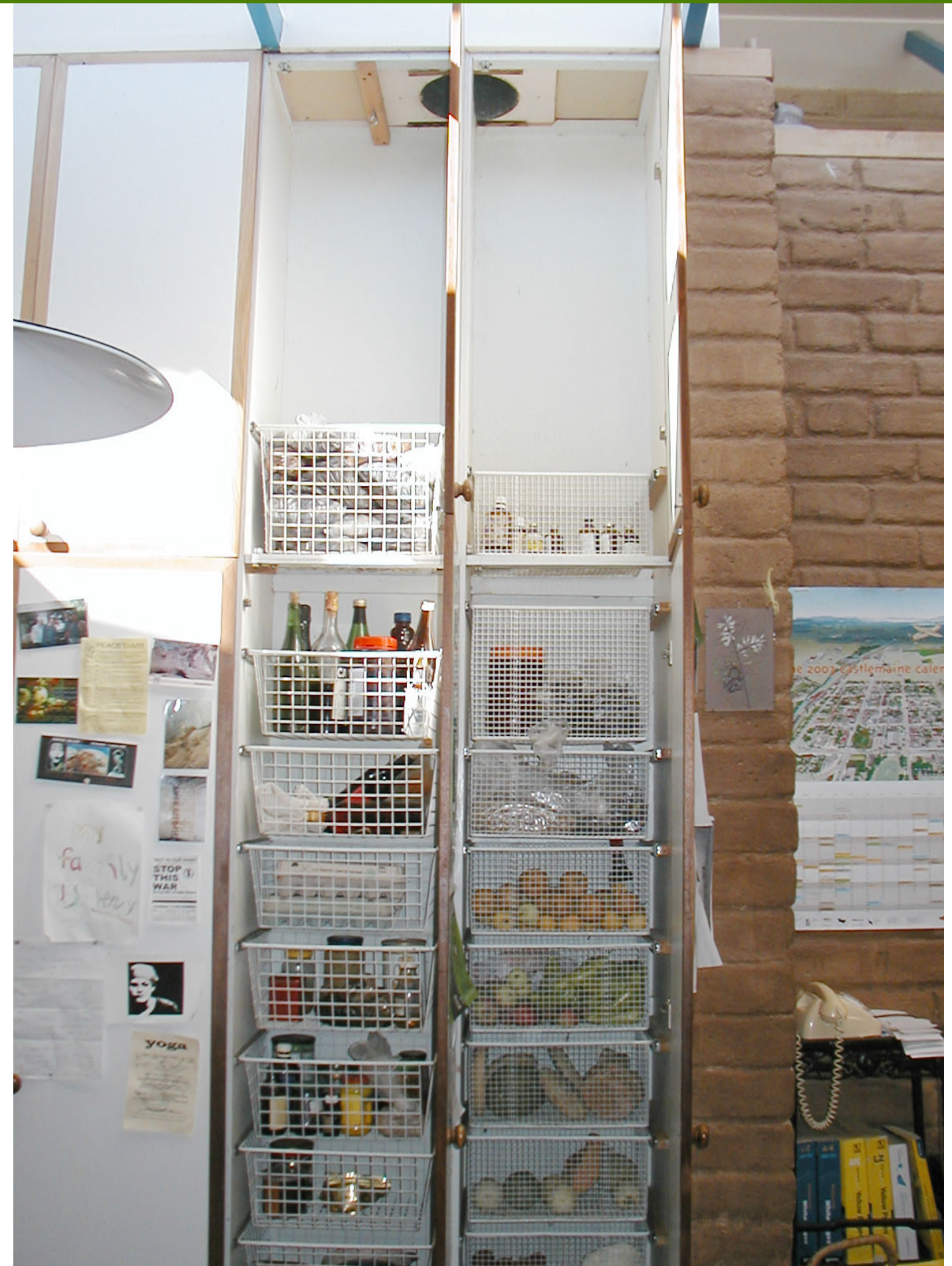
Double column cool cupboard with 300mm diameter metal flue pipe through attic space.
