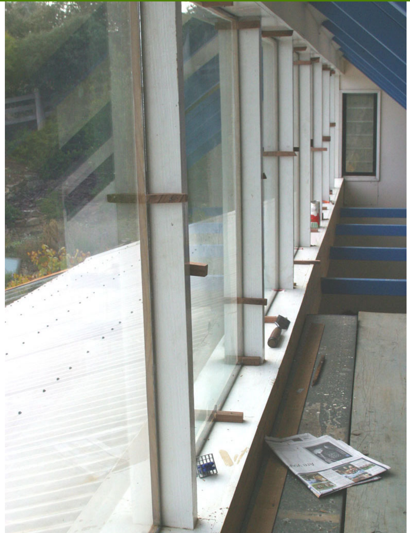
Second sheet of 6mm glass fixed over 10mm bead to form double glazed panel with existing 6mm external glass. Note wooden blocks to clamp glass until silicon sealant dries.
