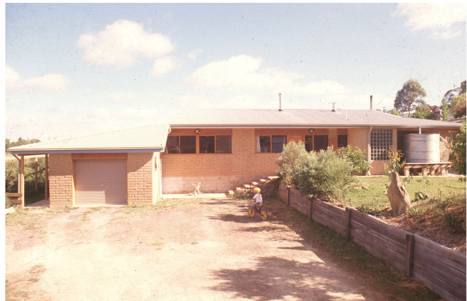
Above: North aspect of house viewed from McKinnon Road reserve winter 1990 showing the large area of north facing glass. Stove flue pipe left, cool cupboard exhaust vent centre, greenhouse exhaust vent lower roof and wood heater flue right. Rabbit proof perimeter fence and rip lines for road reserve plantings in foreground.
