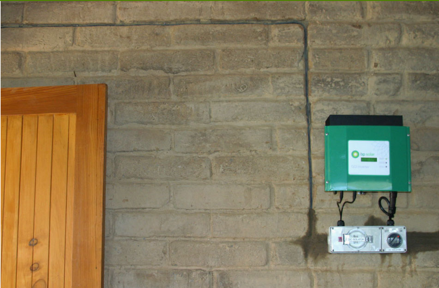
240 volt inverter and isolation switches mounted on mudbrick wall in workshop. Wiring conduit from panels on roof chased into mudbrick. Note fresh mud mortar covering wiring conduit on right leading to meter box switchboard
