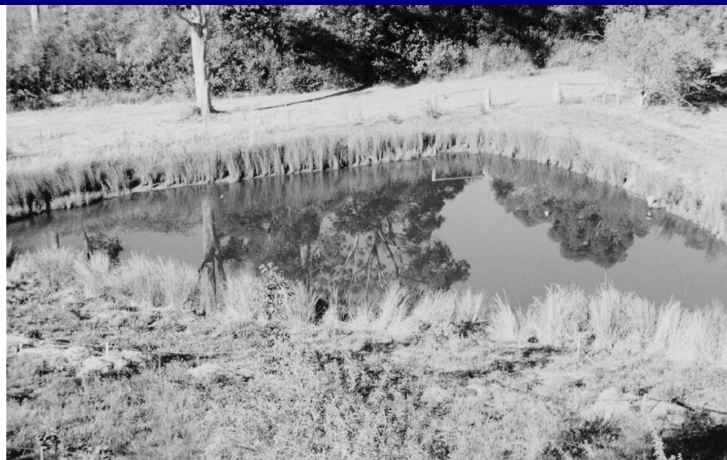
Main dam in early summer 1989 with trickle pipe intake, right, showing 300mm above falling water level from a combination of evaporation and pumping to the header tank for irrigation.
