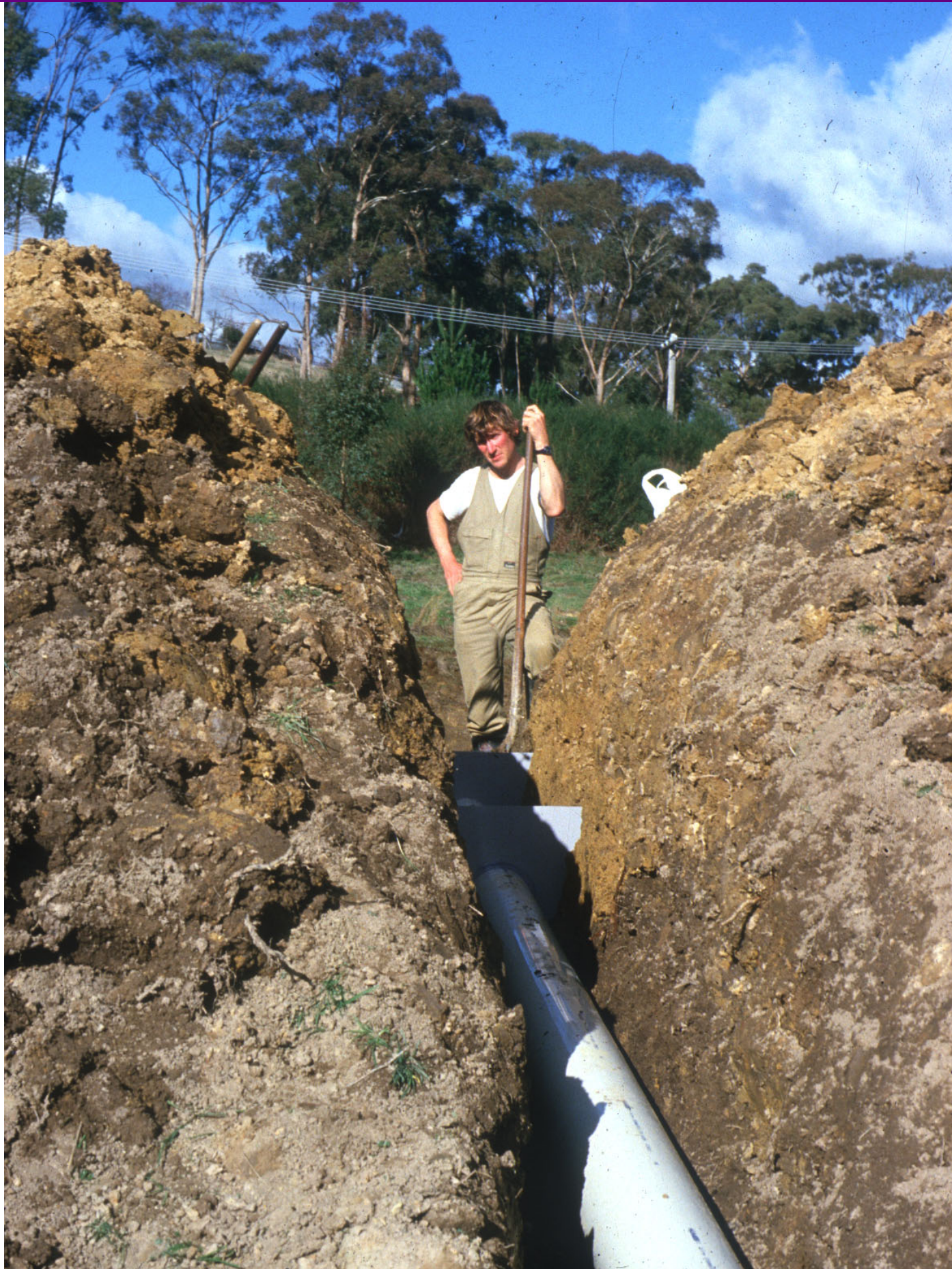
David installing 150mm PVC trickle pipe through main dam wall at the top water level 1987. Two PVC baffle plates prevent seepage along outside pipe.
