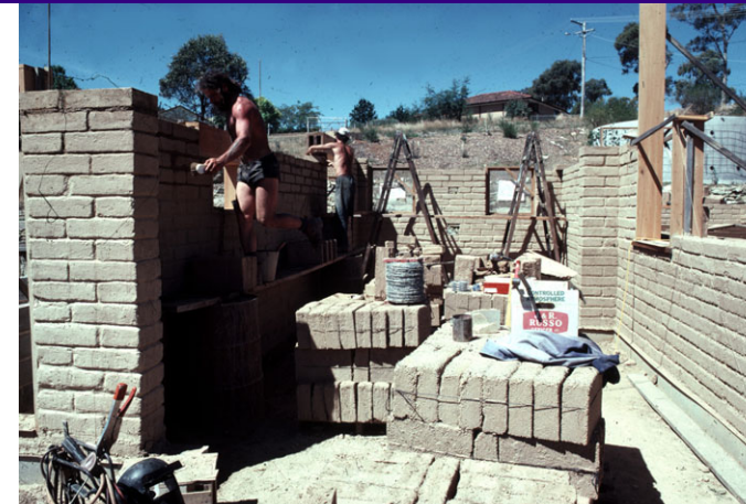
Wayne Irving and Doug Swing laying mudbricks on greenhouse/dining area thermal mass wall. Note boxed beam header above greenhouse-kitchen doorway and steel rods (upper left and centre left) for tie down of timber lintel and roof.
