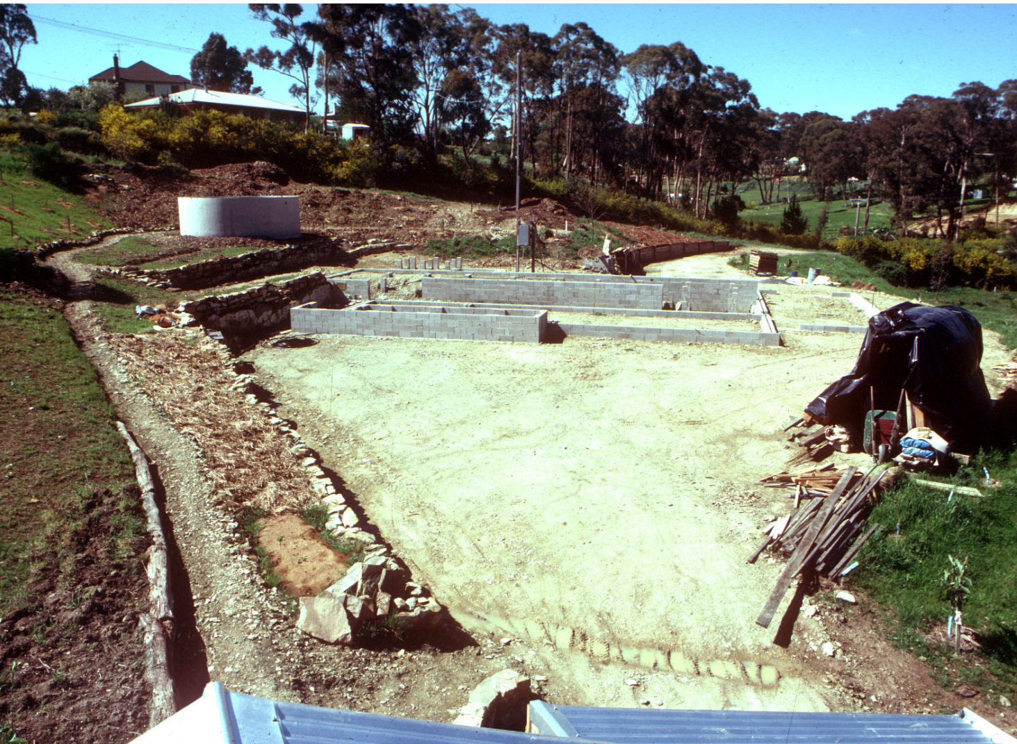
Wide angle view of house site September 1986 from roof of newly constructed shed. Dry stone and timber retaining walls, concrete water tank and house foundation walls, wheelbarrow path, terraces with first mulching over topsoil. Tree planting on fill slope (right) and cut slope (back). Note table drains formed by wheelbarrow path and main platform.
