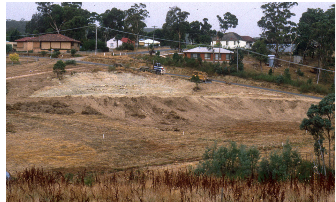
View from Newstead Road of house site excavation completed; split level main platform, tank terrace, fill slope roughly respread with topsoil and topsoil stockpile on left. Stakes in middleground marking out main dam in gully.
