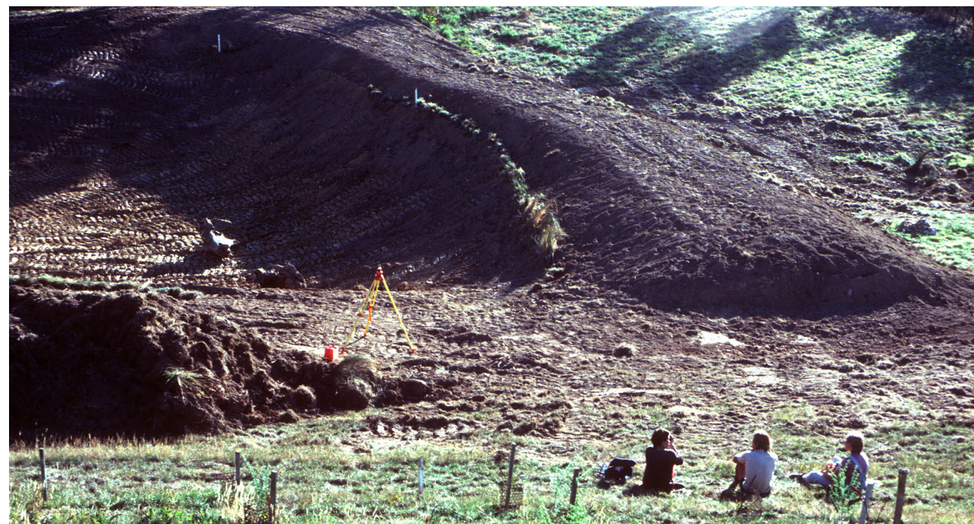
Main dam construction complete March 1987. Topsoil spread on wall and inside slopes. Stakes and Pin rush tussocks mark top water line. Tree stumps in dam for fish habitat, spillway lower right, surplus topsoil stockpile (later moved to housesite garden areas) on left. Tree planting on housesite fill slope in foreground.
