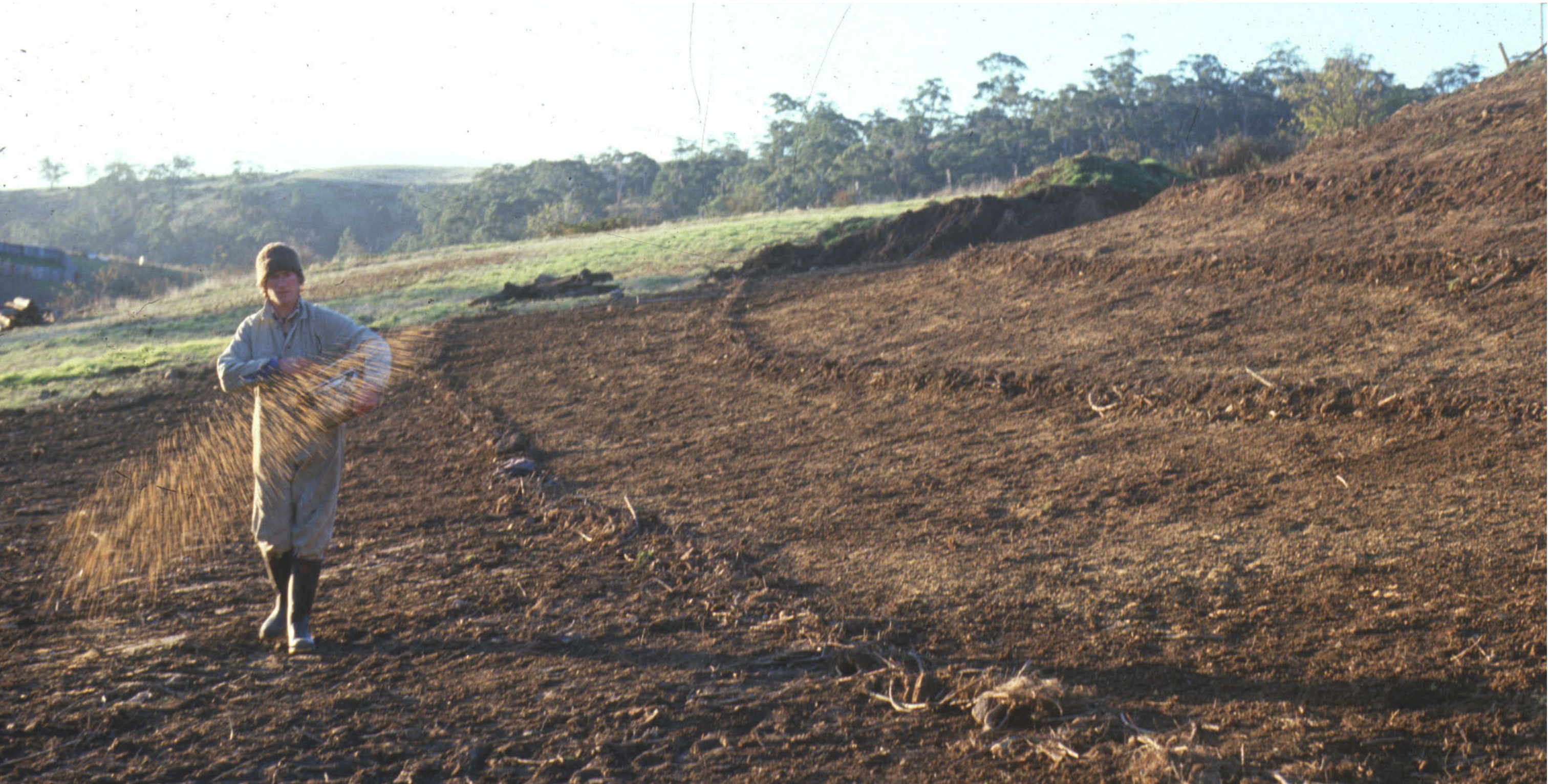
David sowing pasture seed on freshly raked topsoil of fill slope, May 1986. Debris raked to contour lines for erosion control. Topsoil stockpile back right. Species mix; tall fescue, phalaris, cocksfoot, prairie grass, white and subterranean clovers.
