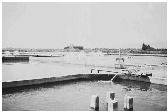
Figure 2. Poured concrete recirculating tanks used for intensive rearing of eels. (Courtesy of G. Degani.)
