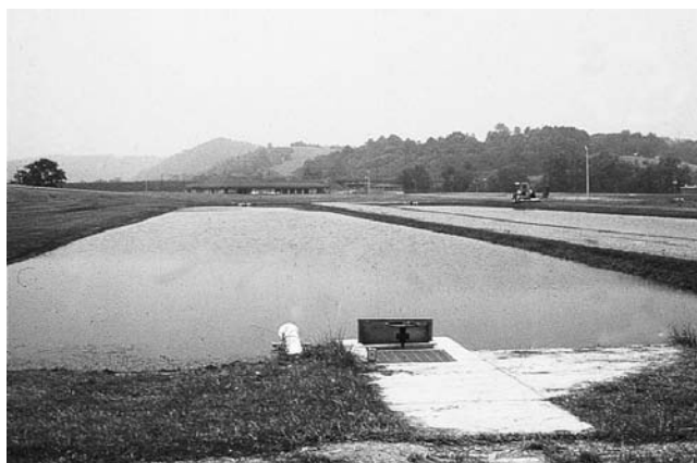
Figure 1. A typical fish culture pond, showing an inflow pipe to the left of the drain structure.
