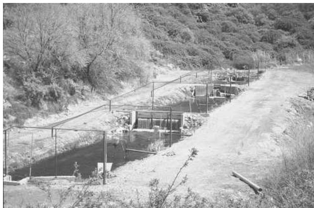
Figure 5. Typical earthen ponds used in Idaho. Note the bird netting to keep birds out.
