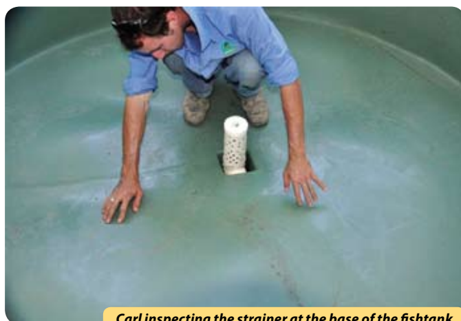
Carl inspecting the strainer at the base of the fishtank
