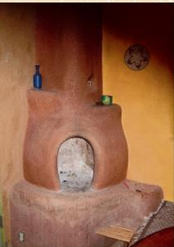
Kitchen fireplace, handcrafted from molded clay, straw and pumice
