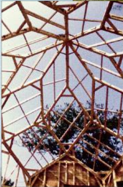
Looking up at interior structure of zome shown in background photo
