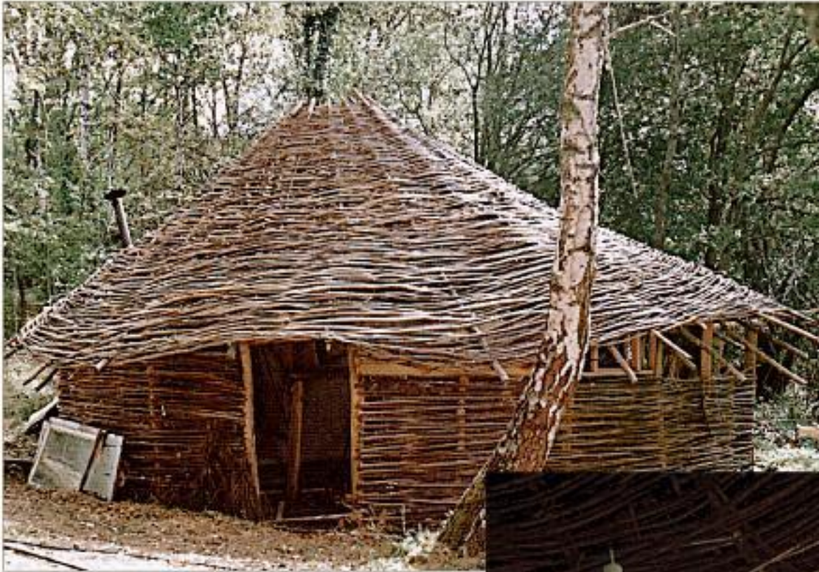
These three photos show stages of building an Arigean yurt for a music studio. Above: Locust and chestnut branches on posts, hazel branches woven horizontally
