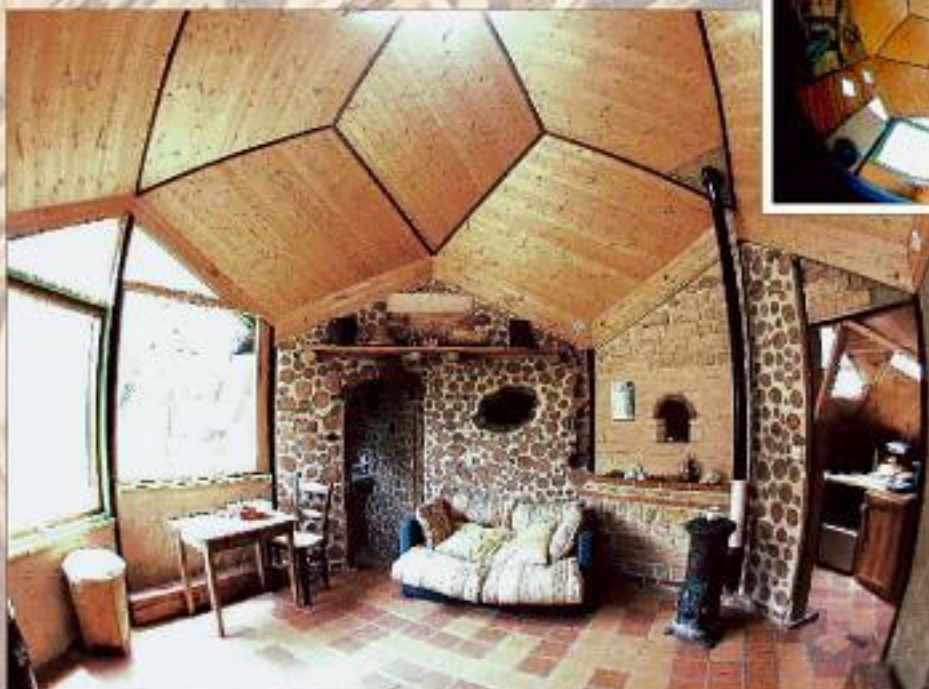
Interior shows use of different materials: adobe, wood, cordwood, cob; it's insulated with sheep wool, straw, and clay.
