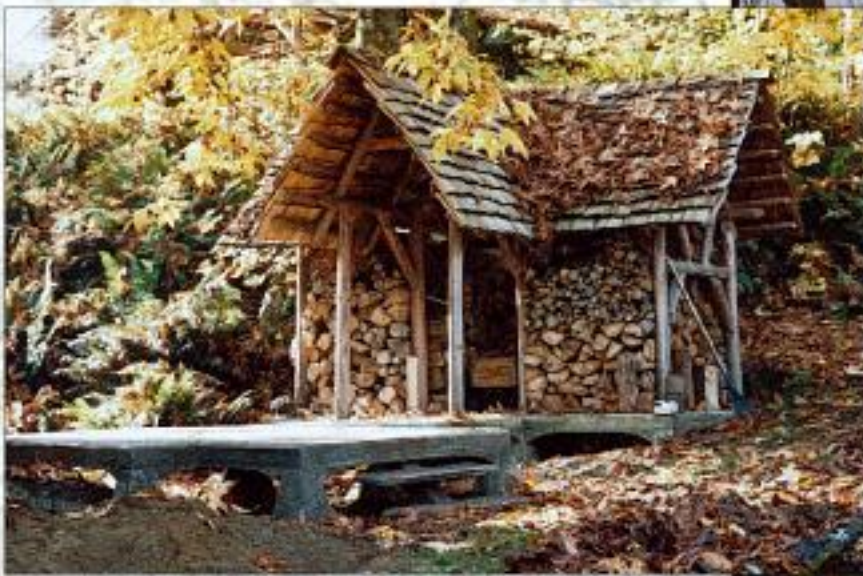
Woodshed ready for winter. Built on 4"-thick edge-supported structural slab with integral steps
