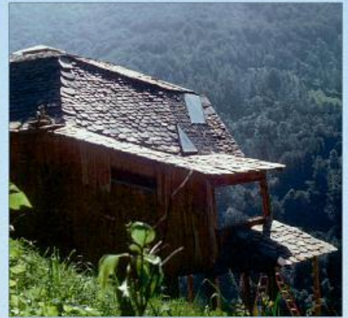
Zome in mountains is roofed with 100-year-old slate shingles obtained from abandoned buildings in the area.
