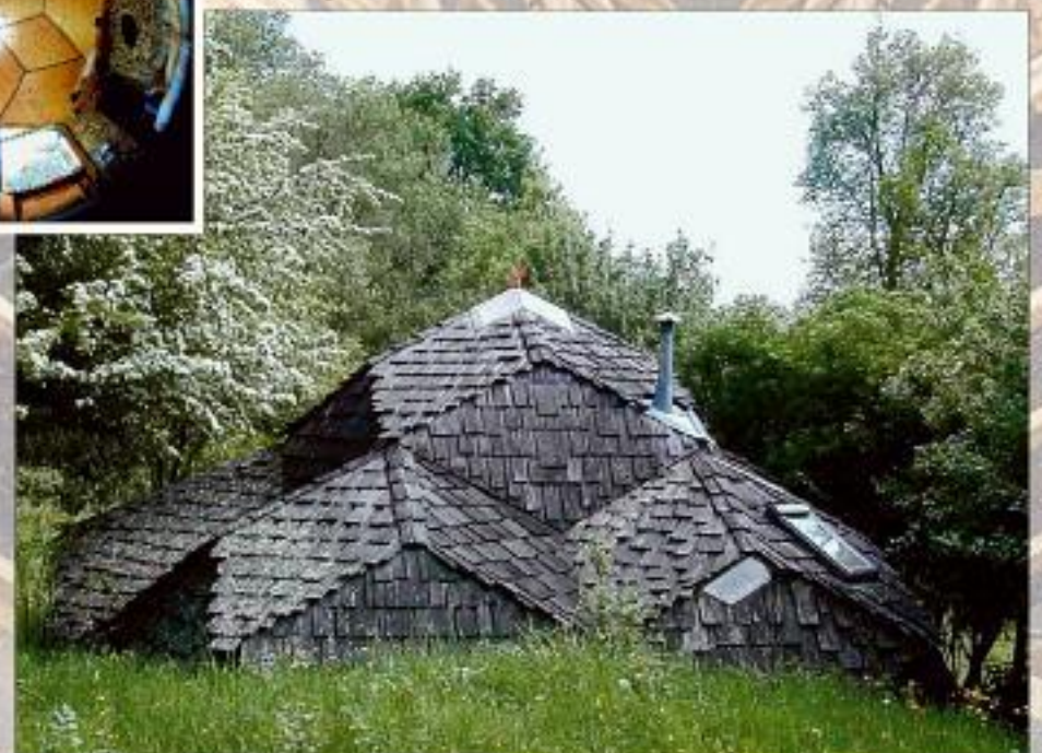
North face; main rhombitriacontahedron is clustered with offshoots of the same geometry, producing wave-like effect.
