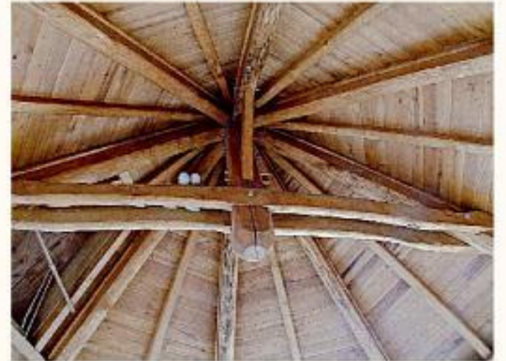
Roof framing of circular cabin
