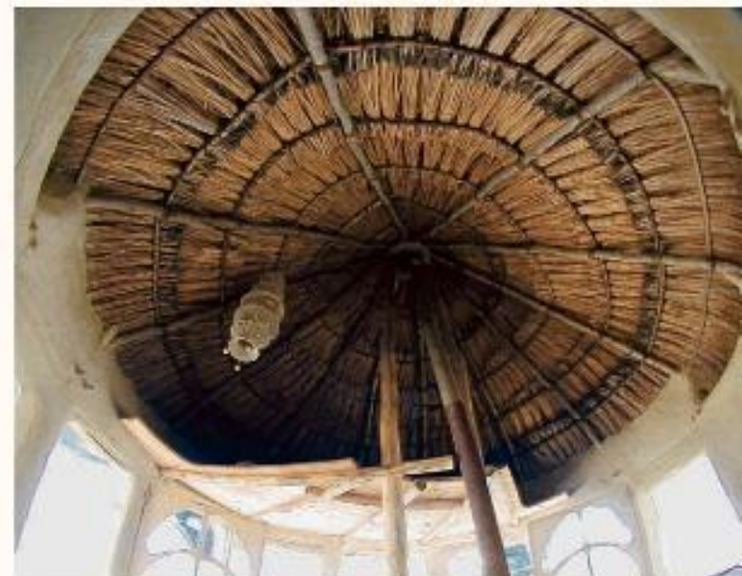
Roof thatched with ferns, visible inside
