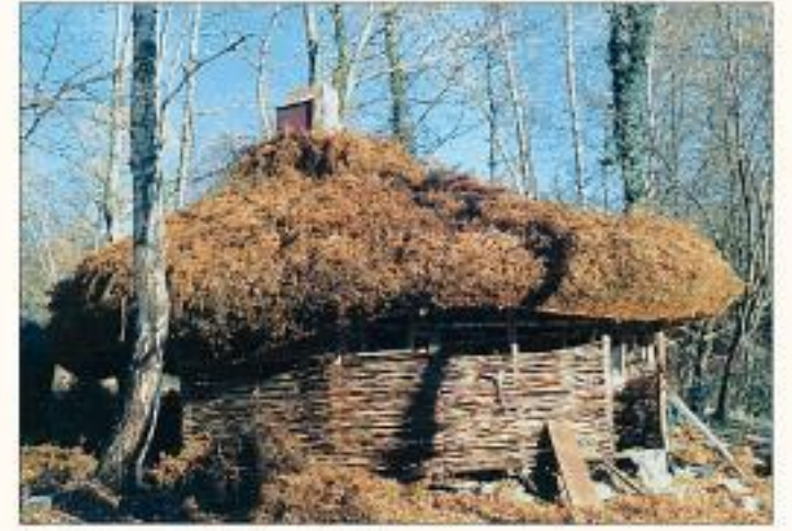
Roof covered with fern thatch
